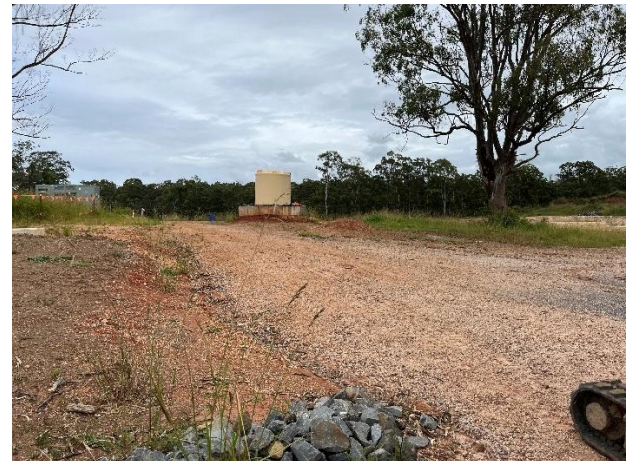
TP5- Looking north along Road 5 Ch40m that is underlain by gravel fill and red residual clay.
