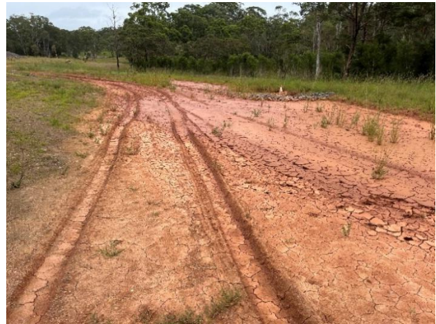
TP2- Looking west along Road 10 Ch75m that is underlain by clay fill.
