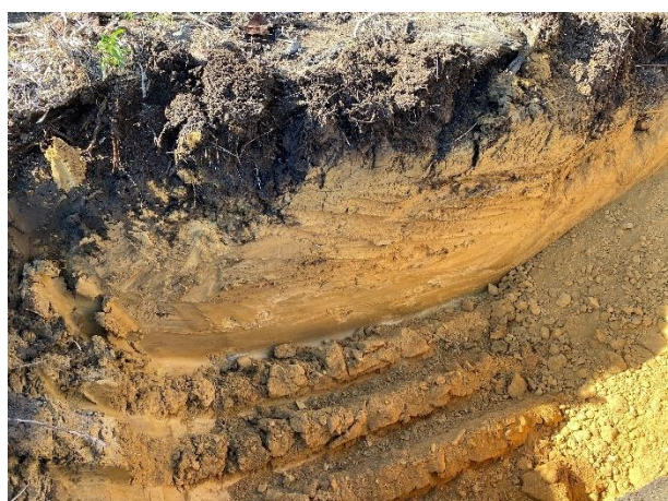
TP2: Pale yellow residual clay (Unit 4B), that is typically highly reactive and low CBR. Generally not suitable for reuse as engineering fill unless blended with weathered rock.
