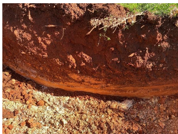
TP4: Orange/red residual clay Unit 4A, typically of medium CBR, overlying white clays (Unit 5A) of typically low CBR that should be stockpiled separately during regrading works.
