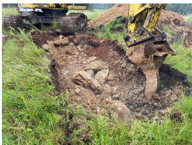
TP-HILL B: Single tyne ripper used to break up band of low strength dolerite rock.
