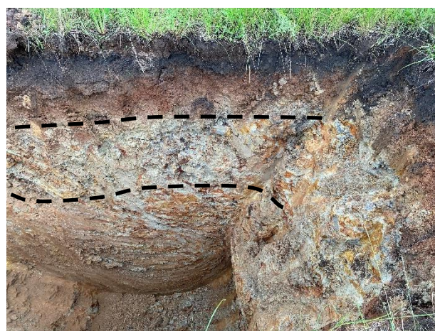
TP-HILL A: Band of highly weathered dolerite rock present from 0.7m to 2m was underlain by clay soils to 5.2m.
