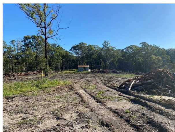
Looking west from TP1. Surface soils disturbed by tree removal and some stump holes are likely to be present.
